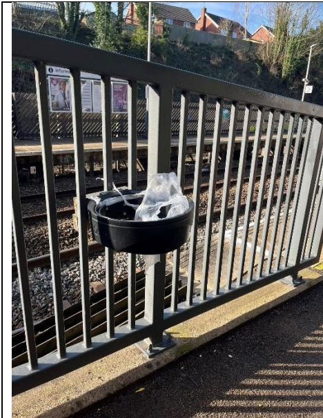
Rubbish bags ripped away
