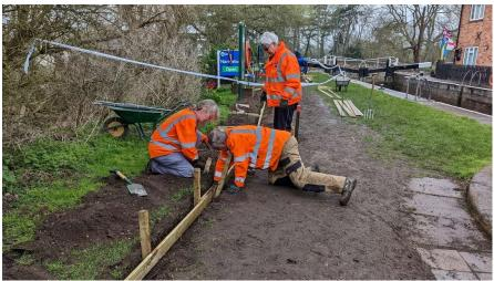
**12**<sup>th</sup> **April** – Lots of gravel – about 12 tonnes was moved by volunteers onto the path alongside completing the last of the shuttering. The 60m stretch also had the whacker plate over it a few times to start to bind the layers of fine gravel together
