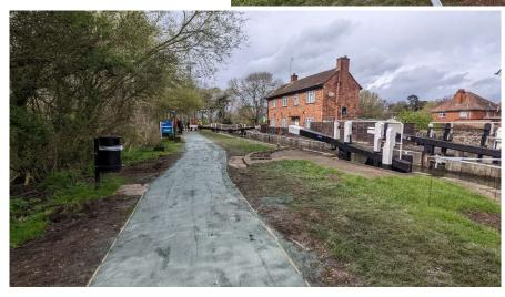
**19<sup>th</sup> April** – After a week of settling, the path had another rake over to try to level off any lumpy patches before the whacker palte went over it for a final time. A few additional flagstones were put in place around areas of heavy usage to try to reduce wear and tear. The soil that was initially distrurbed from around the path edges was put back in place ready for some grass seed.
