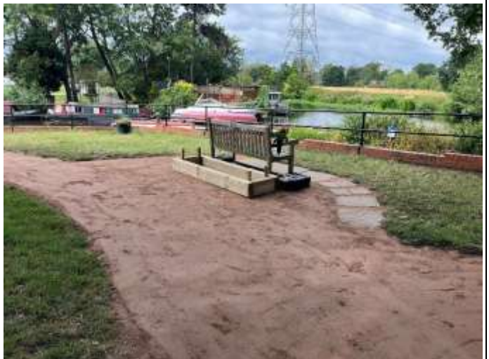
New planter by the memorial bench being installed with new path layout
