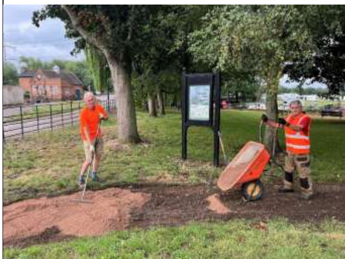
Nick and Brian laying grano on the newly widened path
