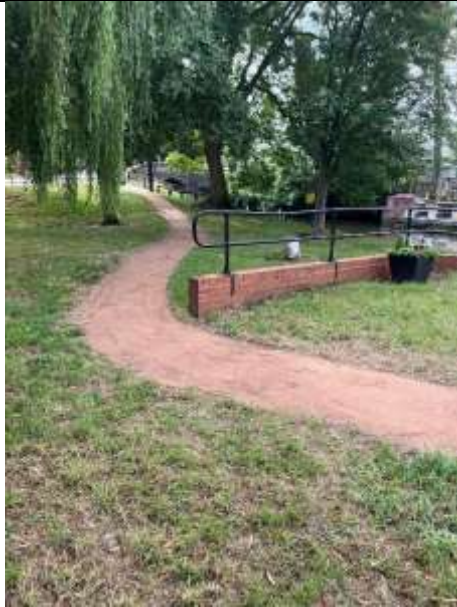
The path up to Deep Lock with a top layer of pink grano to tie into the rest of the area
