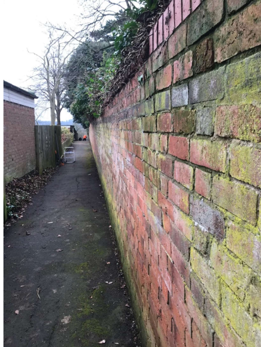
Looking towards Railway - after
