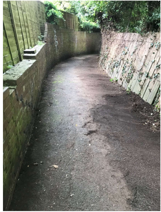
Middle - Looking Down - After
