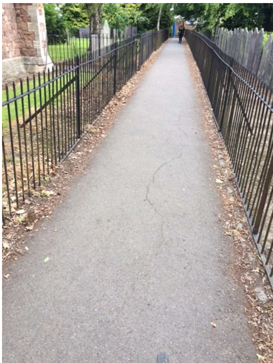
Church Lane - Before
