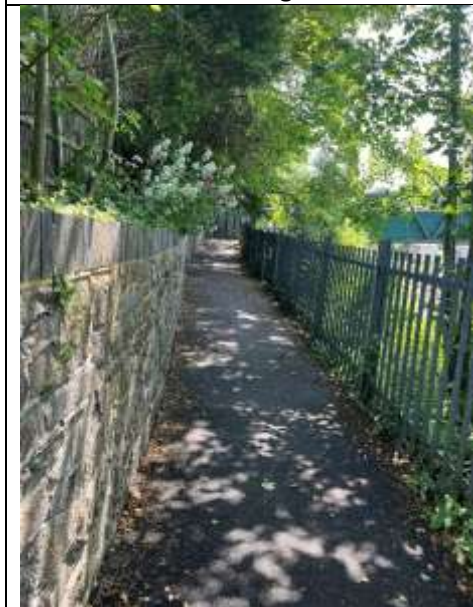
Footpath adjacent to the railway bridge
