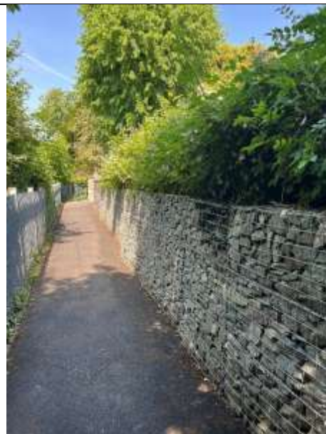
Footpath adjacent to the railway bridge
