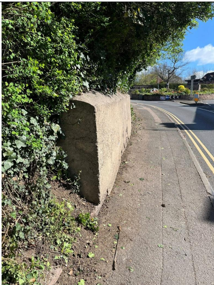
Top of Bridge St cleared
