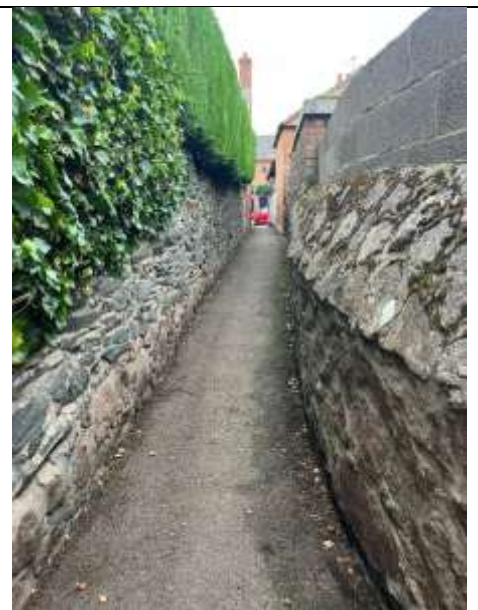
Finally finished -Beveridge St entrance - cleared
