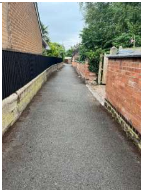
Middle section -towards Beveridge St - cleared
